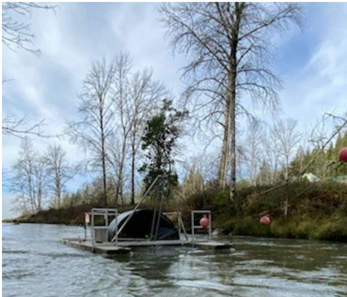
Figure H-17. Lookout Dam Tailrace – Spillway.
