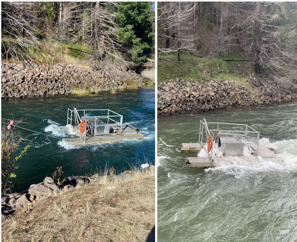
Figure H-9. Cougar Dam – regulating outlet at medium (left) and high (right) flow.
