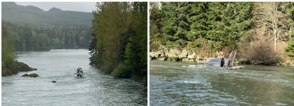
Figure H-18. Lookout Dam Tailrace – Powerhouse Channel in the old orientation where one trap was staggered behind the other (left) and in the new orientation side by side (right).
